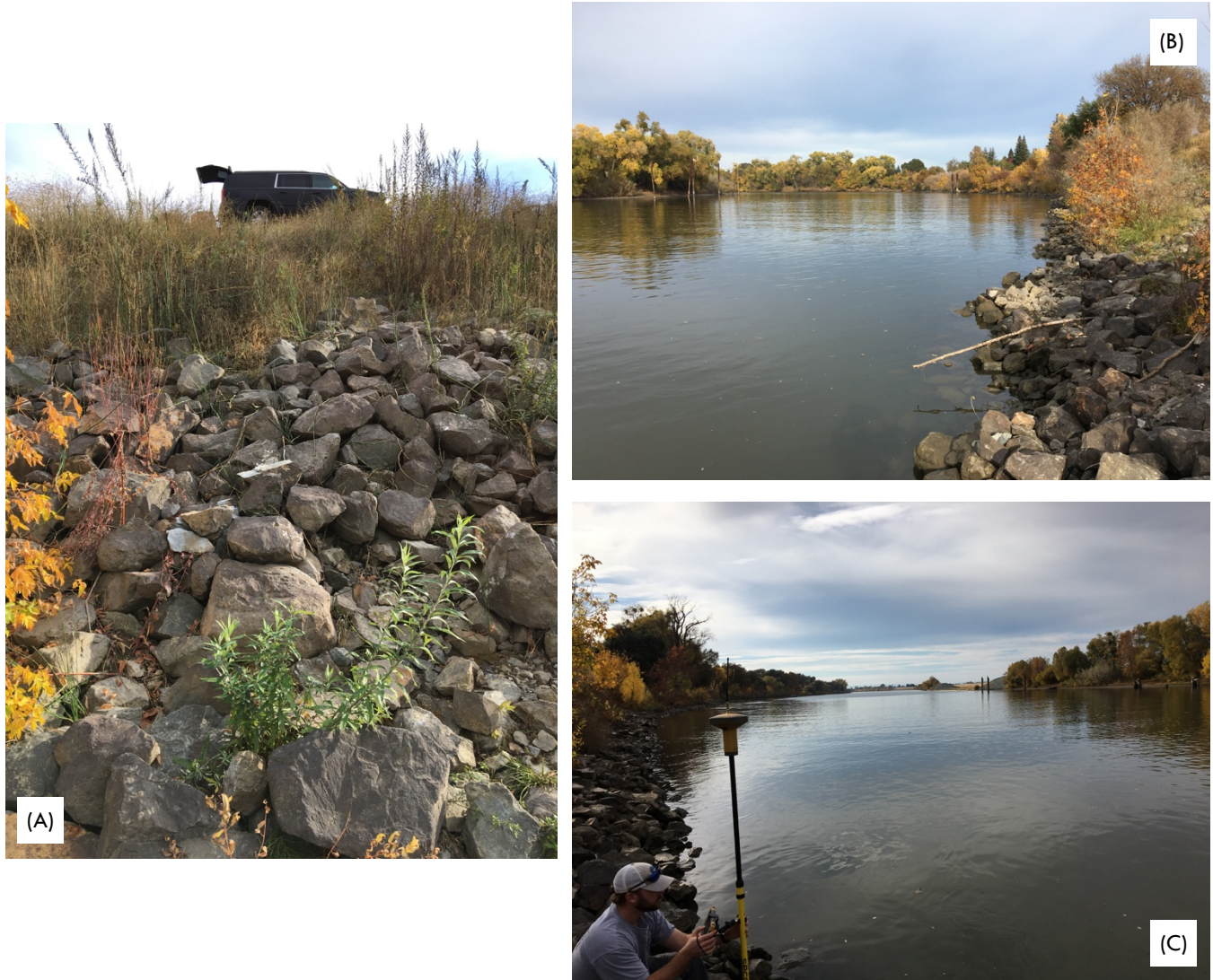
FIGURE 51 – PHOTOS OF STUDY SITE SAC5 ON THE SACRAMENTO RIVER: (A) BANK SURFACE, (B) VIEW UPSTREAM, AND (C) VIEW DOWNSTREAM.
